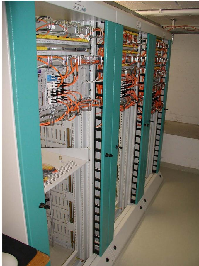
**Figure 17:** In the basement of the WMI a new stacked switch providing 68 fiber optic connectors was installed to switch data packets within the WMI as well as from the WMI to the internet and vice versa.
