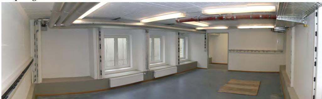
**Figure 2:** Status of the interior work in November 2010. The floor, the windows, the pit in the floor (closed with wooden planks) and the electric lighting is finished. The photo is taken in south-eastern direction from a point similar as in Fig. 1.
