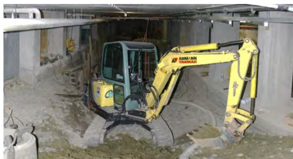
**Figure 1:** Structural work in the basement of the Walther-Meißner-Institute (north-west-corner) in January 2010. Using a suitable digger, the gravel previously filling parts of the basement was removed. The picture is taken in southern direction from the north wall of the building.
