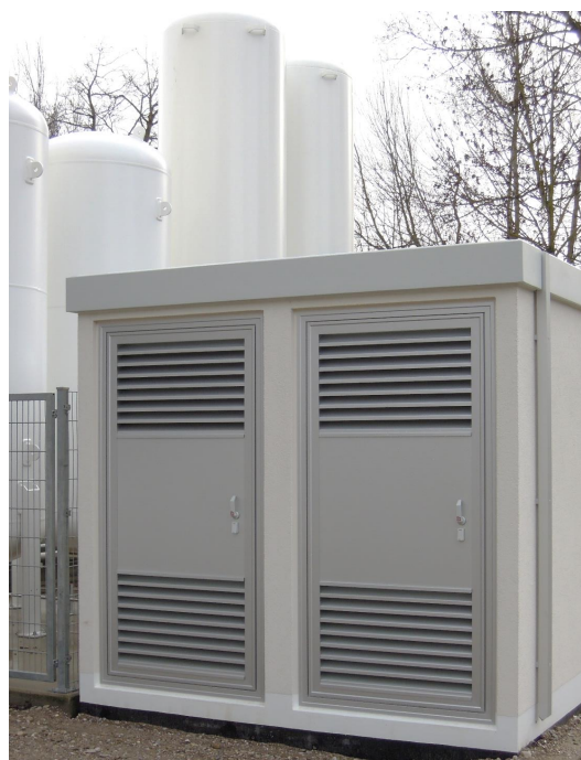
Figure 7: The new transformer station positioned at the south-west corner of the WMI building.
