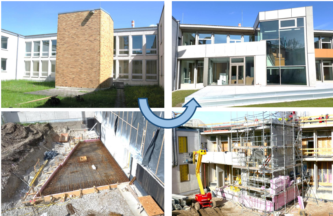
Figure 2: The main staircase of WMI and the cross-aisles at the north side of the WMI building before and after the reconstruction.
