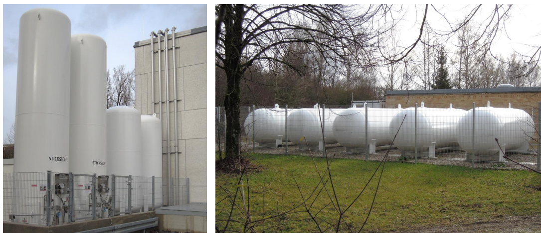
Figure 6: The new liquid nitrogen tanks and new storage vessels for ultra-pure helium gas (left) as well as the new high pressure storage containers for the recovered helium gas (right).
