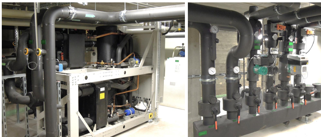
Figure 5: The new refrigerating compressor installed in the basement of the WMI building (left) and the cooling water distribution system (right).
