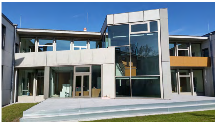
Figure 1: View on the northern cross-aisle and new main staircase of the WMI building as seen from the inner courtyard.
