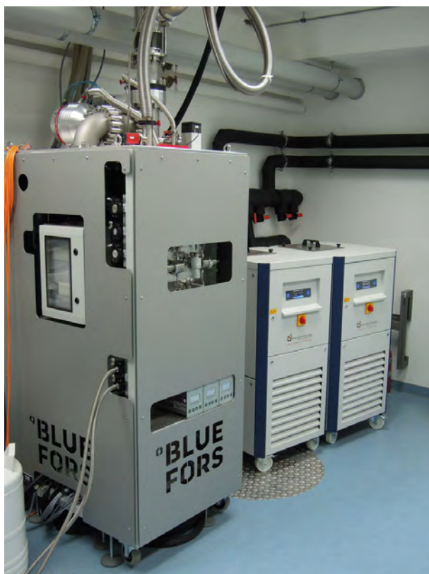
Figure 1: Gas handling cabinet of the Bluefors XLD 1000 system (left) and heat exchangers for the cooling system of the two compressors (right) located in a technical room in the basement of WMI.
